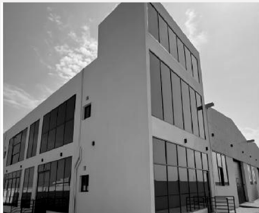
Three-storey administration and engineering block on the factory site
